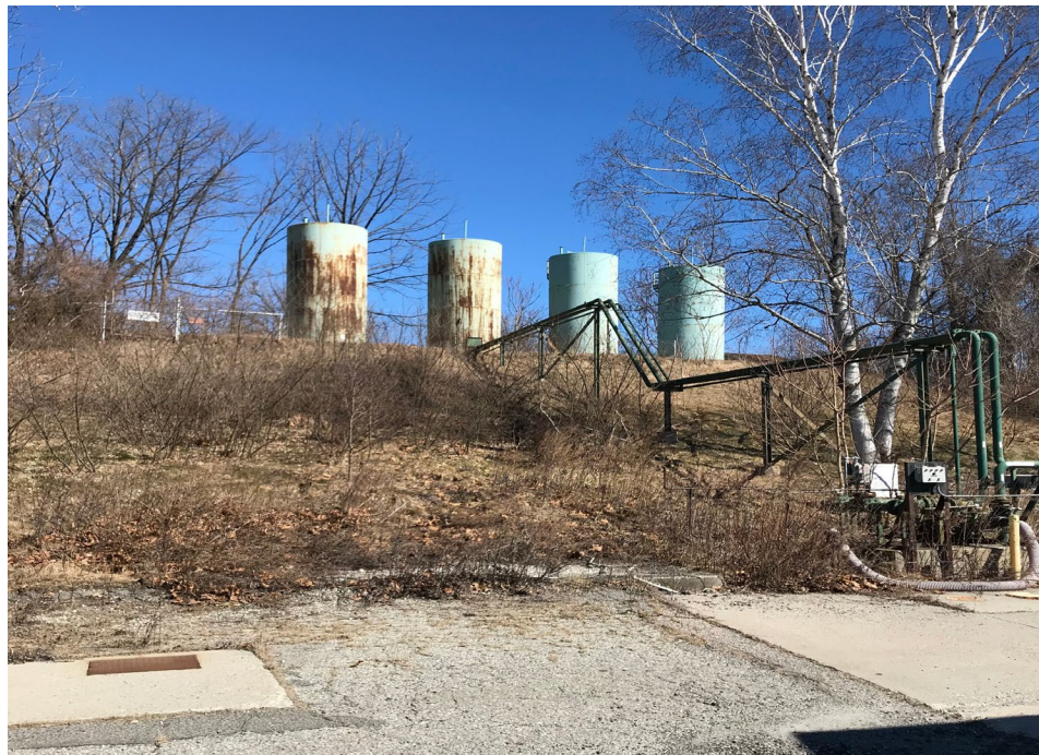
Photograph 7. 8 Young's Field Road's ASTs and pipes connecting them to the western portion of the parcel.
